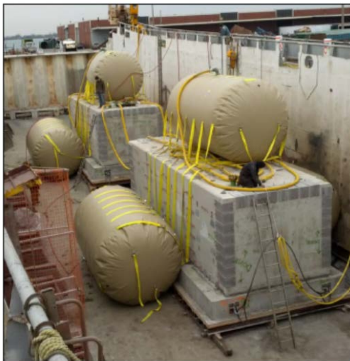
Figure 5.6 Rigid underwater storage vessels used in Hydrostor’s Toronto project being prepped with flotation’s units [Wanwalleghem, 2014]
