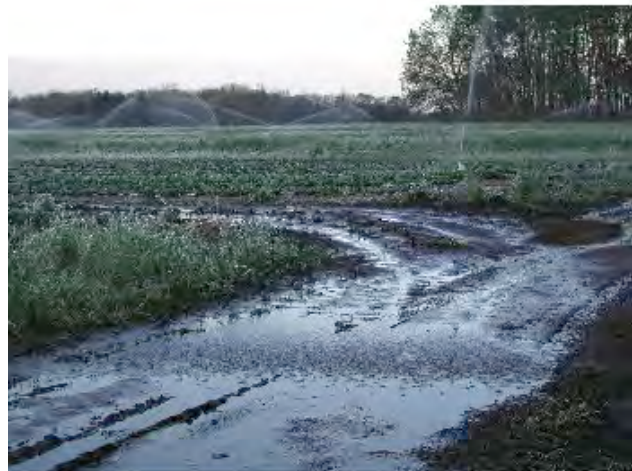
Figure 7a: Standing water and water-saturated soil in a strawberry field
