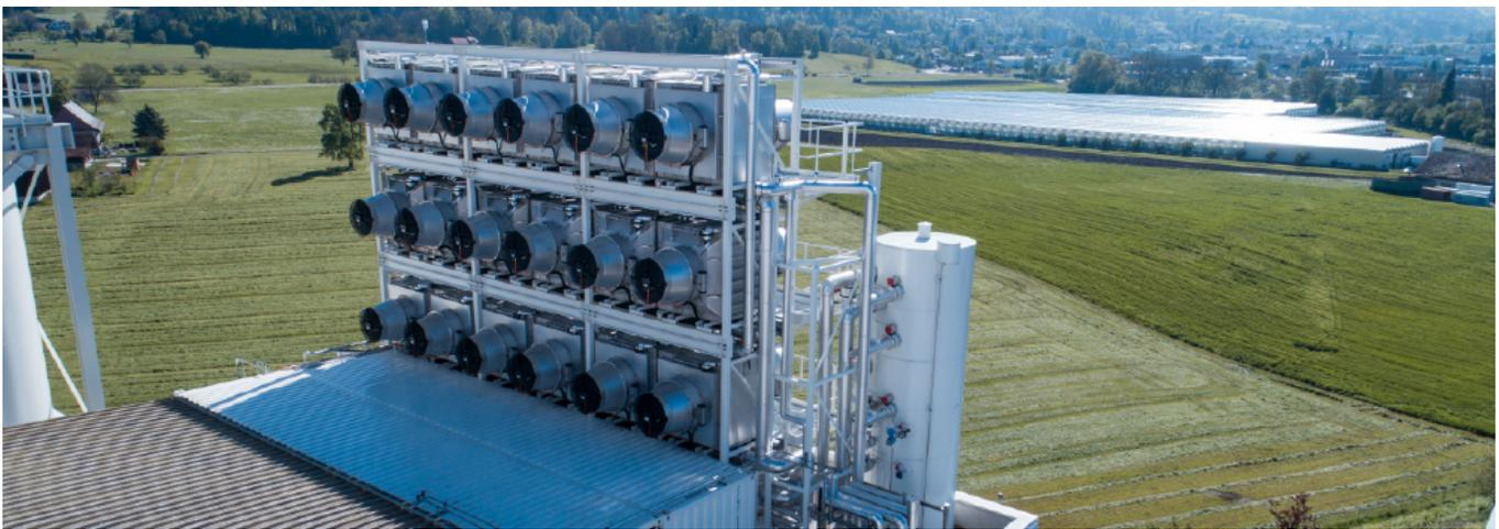
The system consists of a tall bank of fans which draw ambient air in, and through reusable chemical filters which capture the CO<sub>2</sub>. Filters saturated with CO<sub>2</sub> release it for storage when exposed to waste heat from a nearby trash incinerator operation. The CO<sub>2</sub> collected by the system is pure and free of pollutants making it useful for beverage-making, manufacture of synthetic fuels, and other industrial uses.
