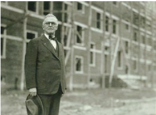
President Hugh Potter Baker, in front of dorm construction, 1940s.
