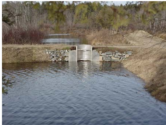
Flume with riprap
