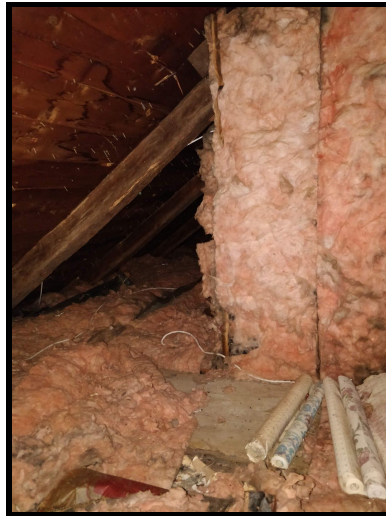
Figure 3.15: Boulder Farm Attic crawlspace
