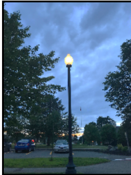
Figure 3.27: These street lights represent one example of indiscriminate outdoor lighting on campus, causing unnecessary light pollution by emitting light in all directions, rather than directing their beams on the intended area below.
