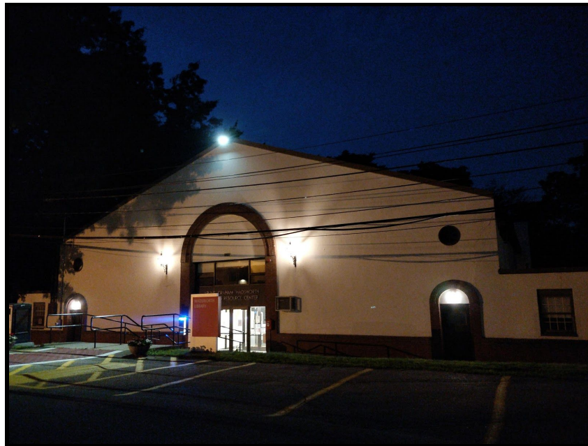
Figure 4.6: Photo of Wadsworth Library exterior lighting and glare
