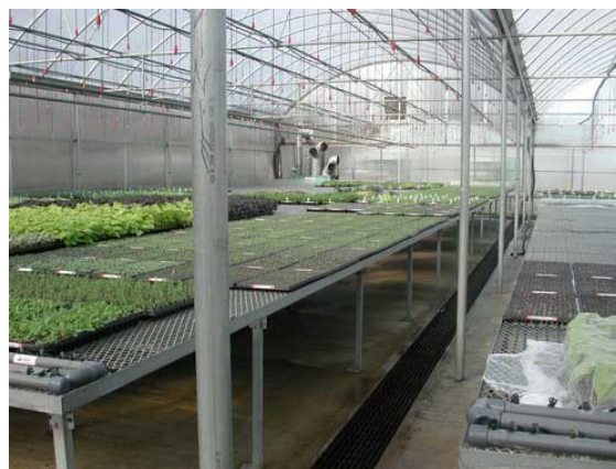
Heated Bench System for Propagation in Gutter-connected Greenhouse
