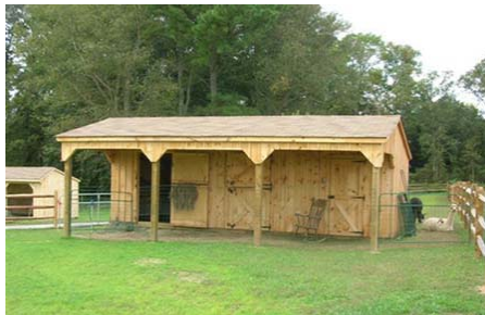
Wooden Lean To Shed
