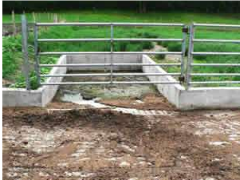
Runoff settling basin
