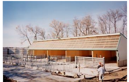
Figure 3. Open sided, single slope roof shed is one of the most common housing structures.
