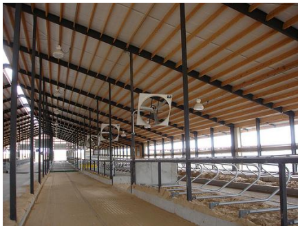
Figure 7. A freestall barn with proper ventilation and fans for air movement.
