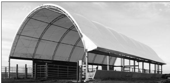
Figure 2. A hoop barn is one of the least expensive structures for housing.
