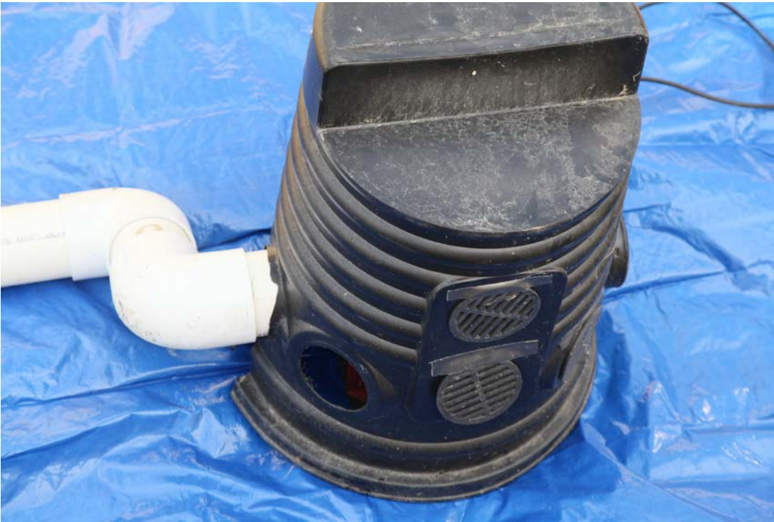
Figure 9. Cover blower to protect from elements.
