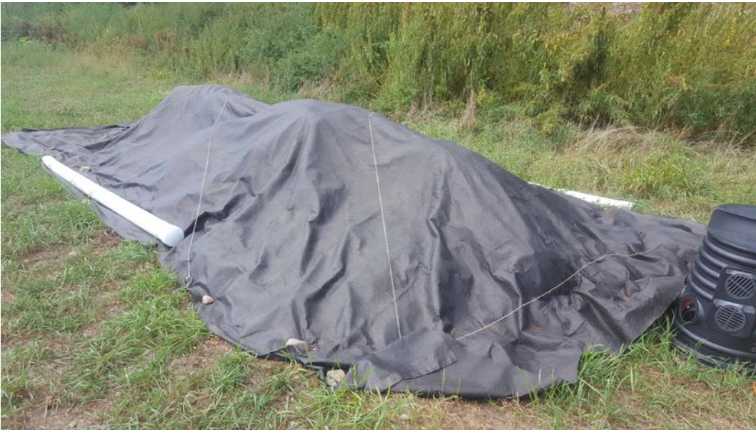
Figure 6. Cover with a geotextile fabric and secure with ropes
