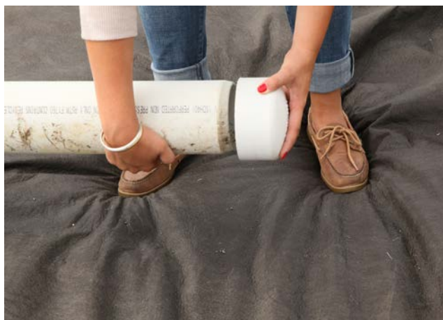
Figure 1. Put cap at one end of PVC pipe.
