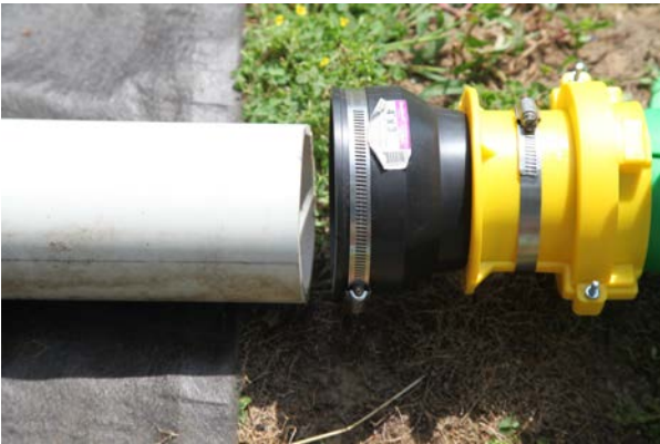
Figure 4. Connect coupling and blower to PVC pipe.
