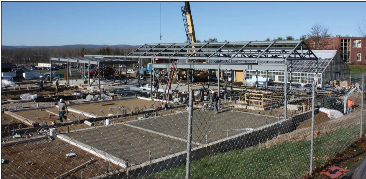
The steel framework of the new headhouse was erected November 23 as work continued on the foundations and floors of the new greenhouses. This view looks north toward Bowditch Hall and original greenhouse in the background.
