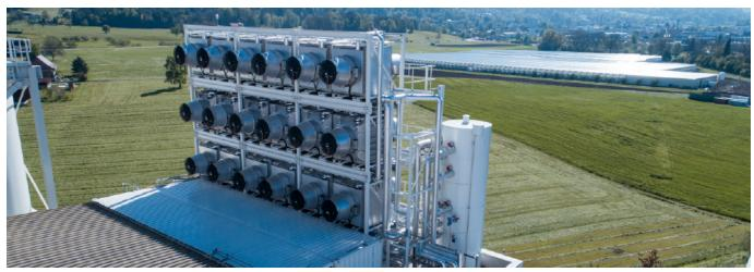
The system consists of a tall bank of fans which draw ambient air in, and through reusable chemical filters which capture the CO<sub>2</sub>. Filters saturated with CO<sub>2</sub> release it for storage when exposed to waste heat from a nearby trash incinerator operation. The CO<sub>2</sub> collected by the system is pure and free of pollutants making it useful for beverage-making, manufacture of synthetic fuels, and other industrial uses.
