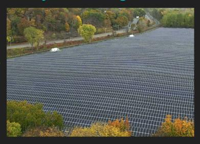
The facility generates approximately 7,300 megawatt-hours of solar energy production which is enough to power 1,800 homes in the area for an entire year.
