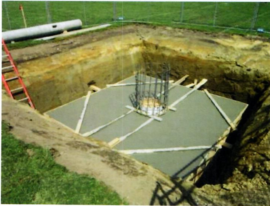
Figure 36. Steel Reinforcing Cage Placed in Center of Footing for Pedestal.
