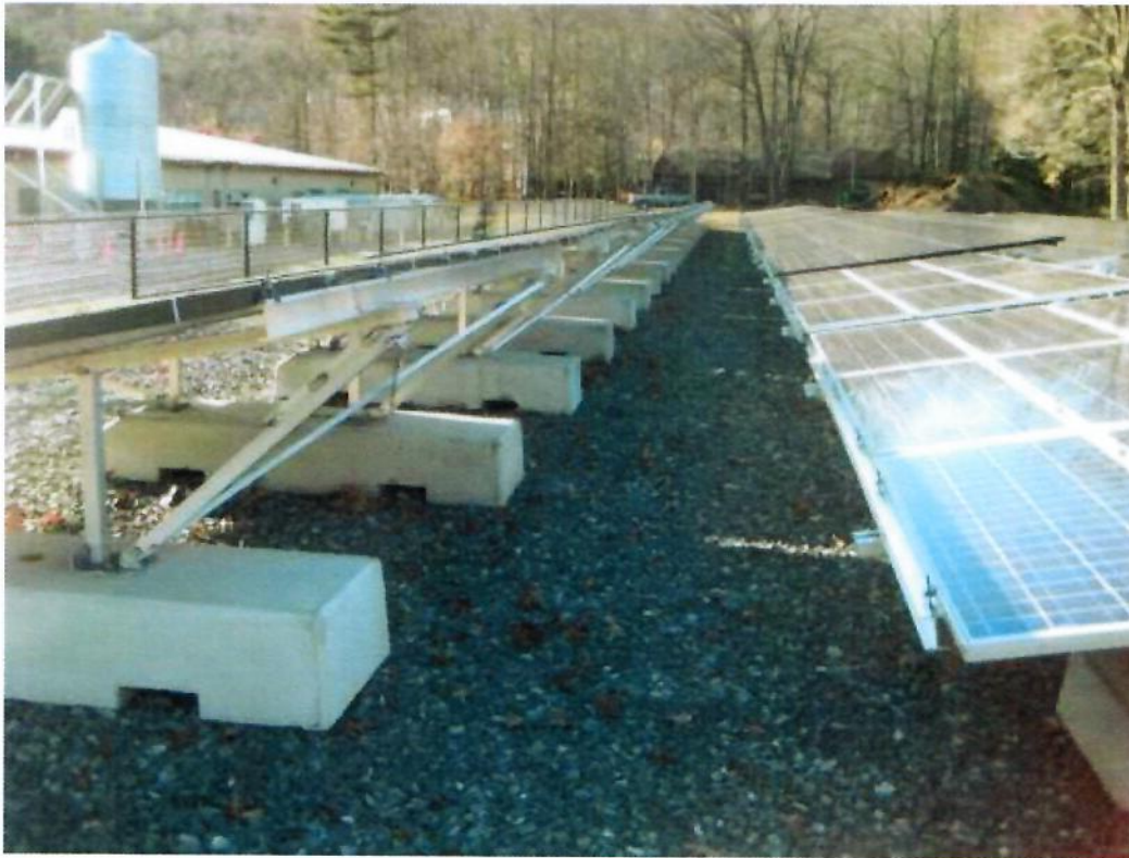
Figure 80. Ballasted Support Using Precast Concrete Blocks – Northfield, Ma.
