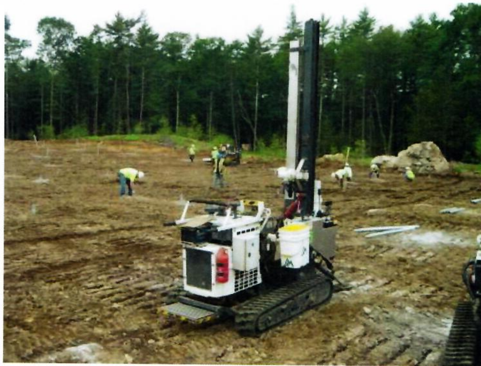
Figure 79. Track Mounted Equipment Used to Install Ground Screws- Sturbridge, Ma.
