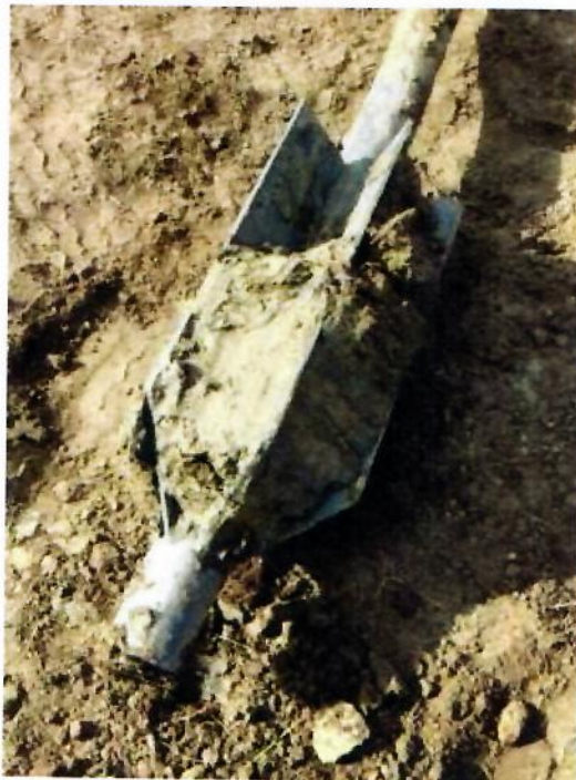
Figure 59. Soil Lodged Between Fins of 6 Fin Pile Extracted from UMass Horse Farm Site.
