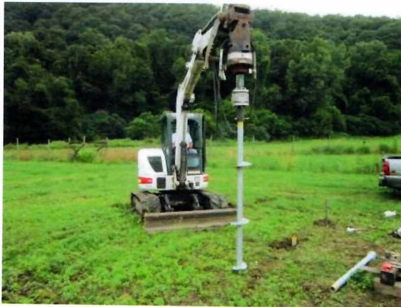
Figure 68. Installation of Helical Piles Using a Compact Excavator.
