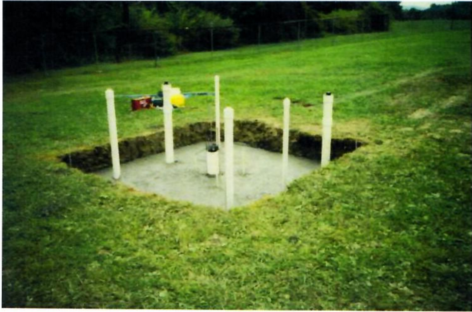
Figure 39. Example of a Neat Excavation for a Cast-in-Place Footing.
