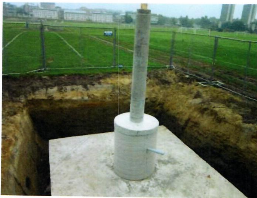
Figure 37. Completed Pedestal and Stem for Cast-in-Place Footing.
