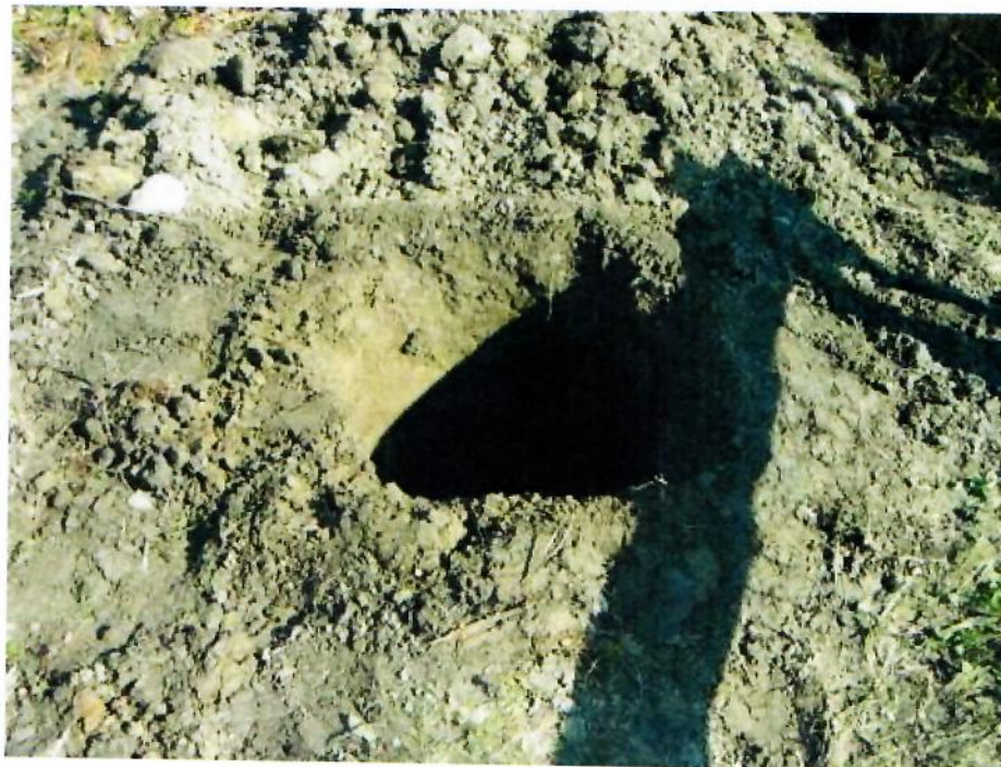
Figure 24. Oversize Drilled Hole for Pedestal Foundation.
