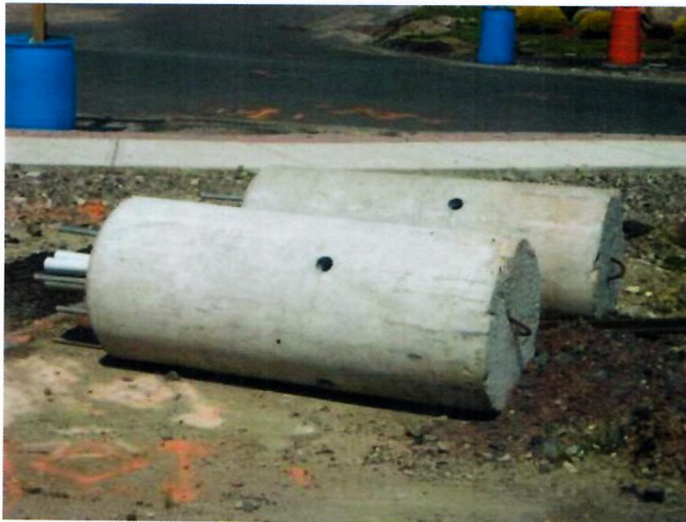
Figure 30. Cylindrical Precast Pedestal Foundation.
