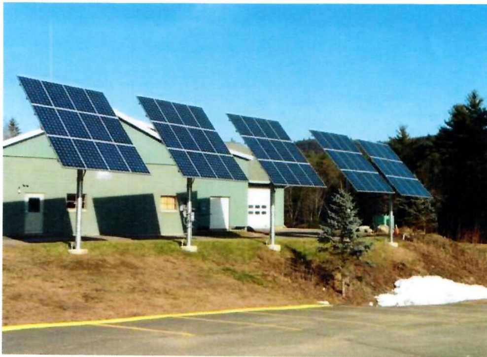
Figure 12. Drilled Concrete Pier Supported PV System, Leverett, Ma.
