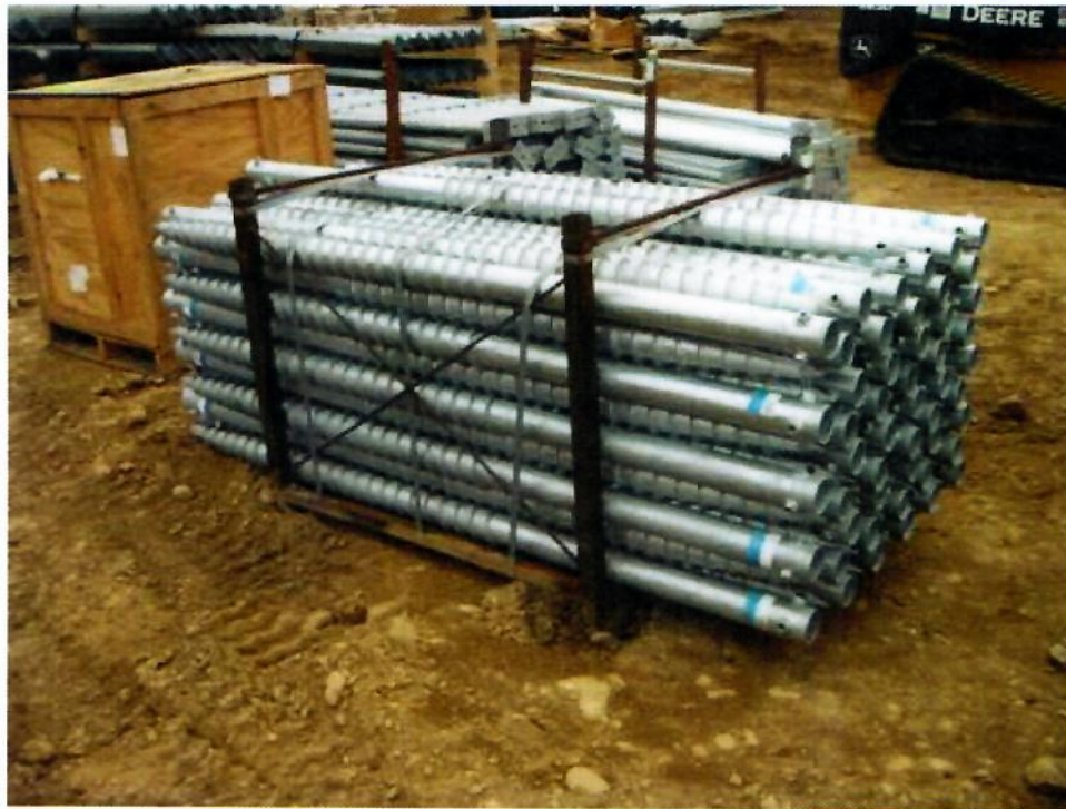
Figure 78. Ground Screws Delivered to a Site to Support PV Panels.
