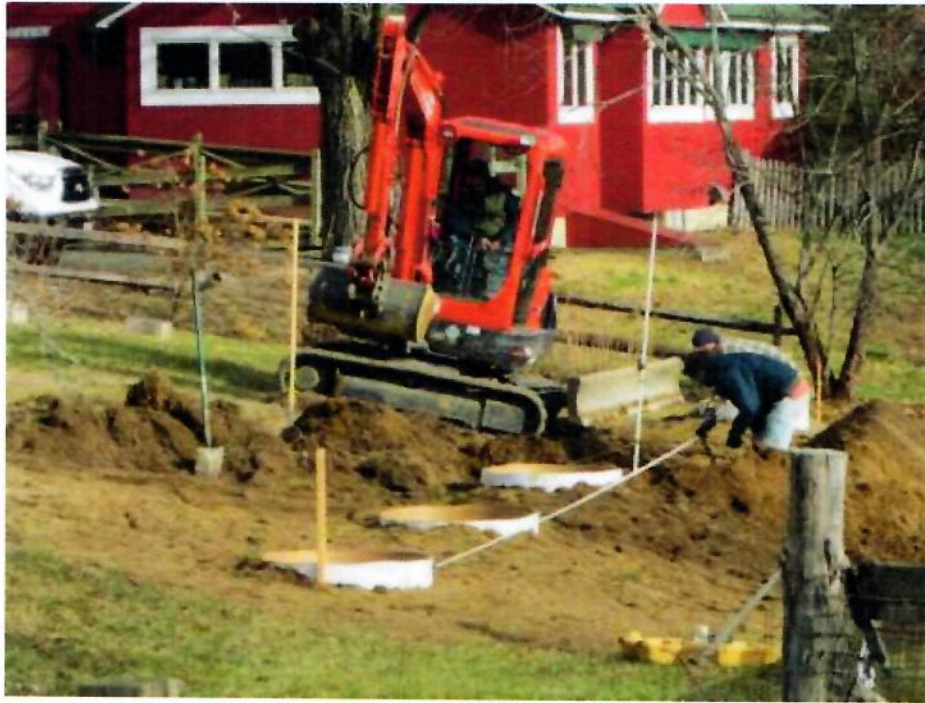
Figure 8. Sonotubes Set For Placing Concrete.
