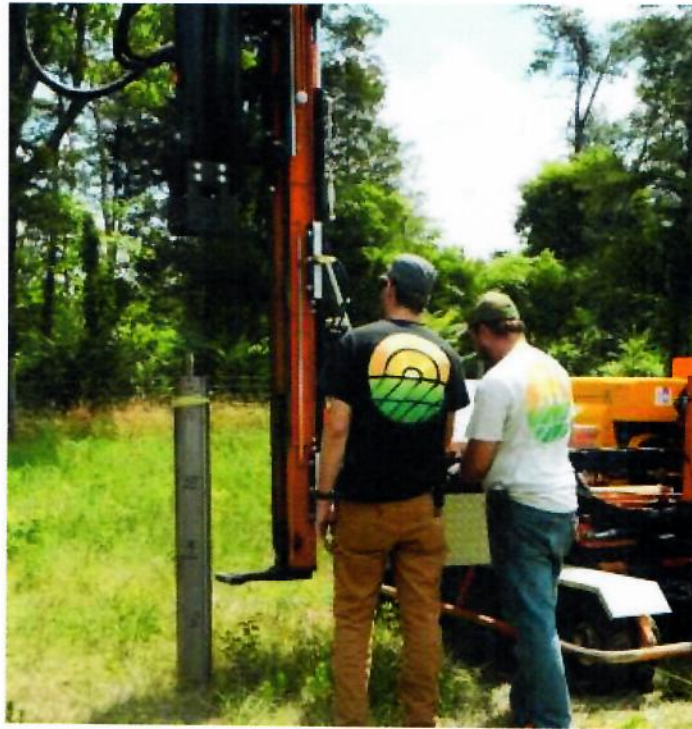
Figure 44. Installation of Steel Piles Using a Special Pile Hammer System.
