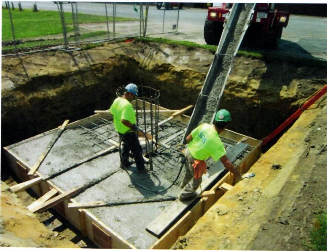
Figure 35. Placing Concrete in a Form for a Shallow Cast-in-Place Footing.
