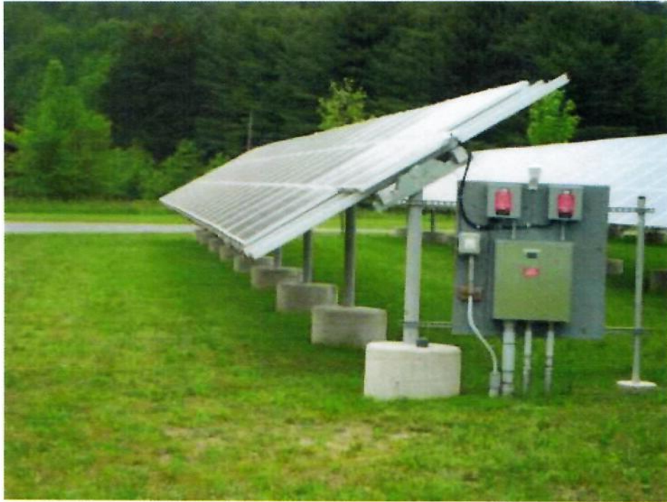
Figure 11. Drilled Concrete Pier Supported PV System - Putney, Vt.
