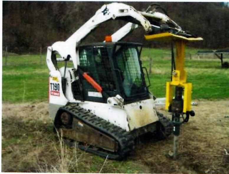
Figure 69. Using a Small Skid Steer to Install Helical Piles.
