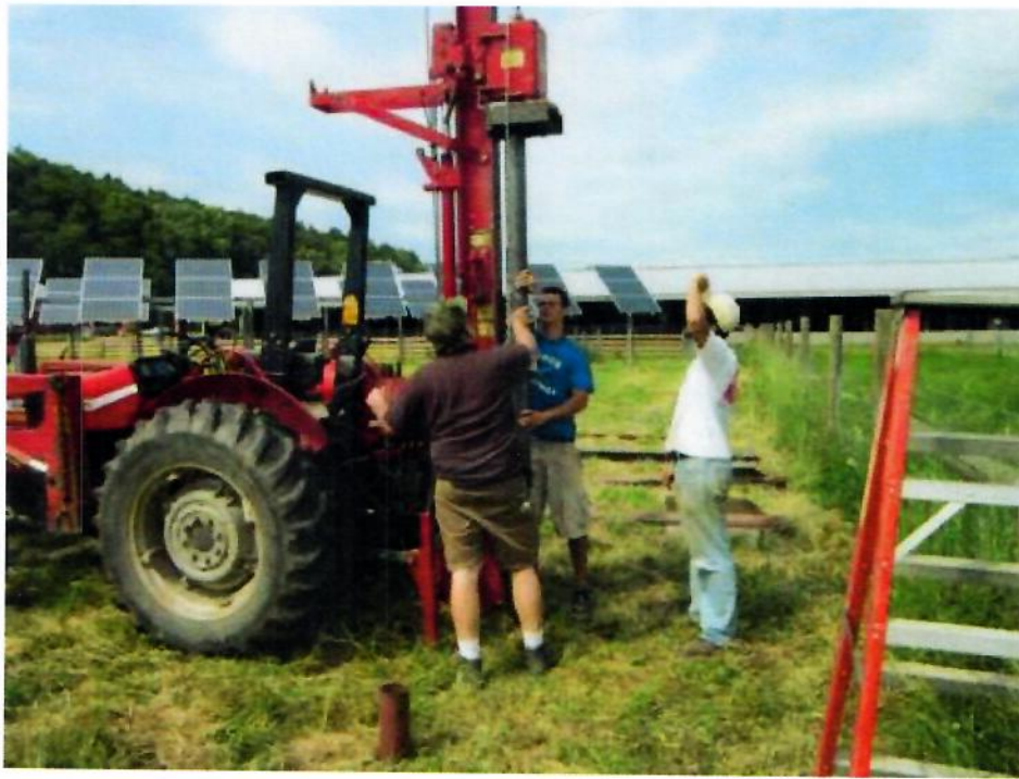
Figure 41. Installing Steel Pipe Piles Using a Tractor Mounted Drop Hammer.
