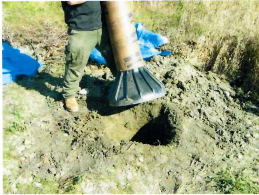
Figure 25. Placing an Enlarged Base Form in Overdrilled Hole for Pedestal Foundation.
