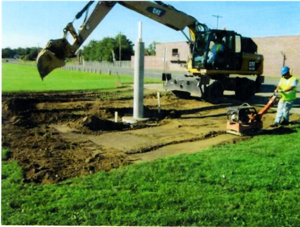
Figure 38. Backfill and Compaction Over the Top of Cast-in-Place Footing.
