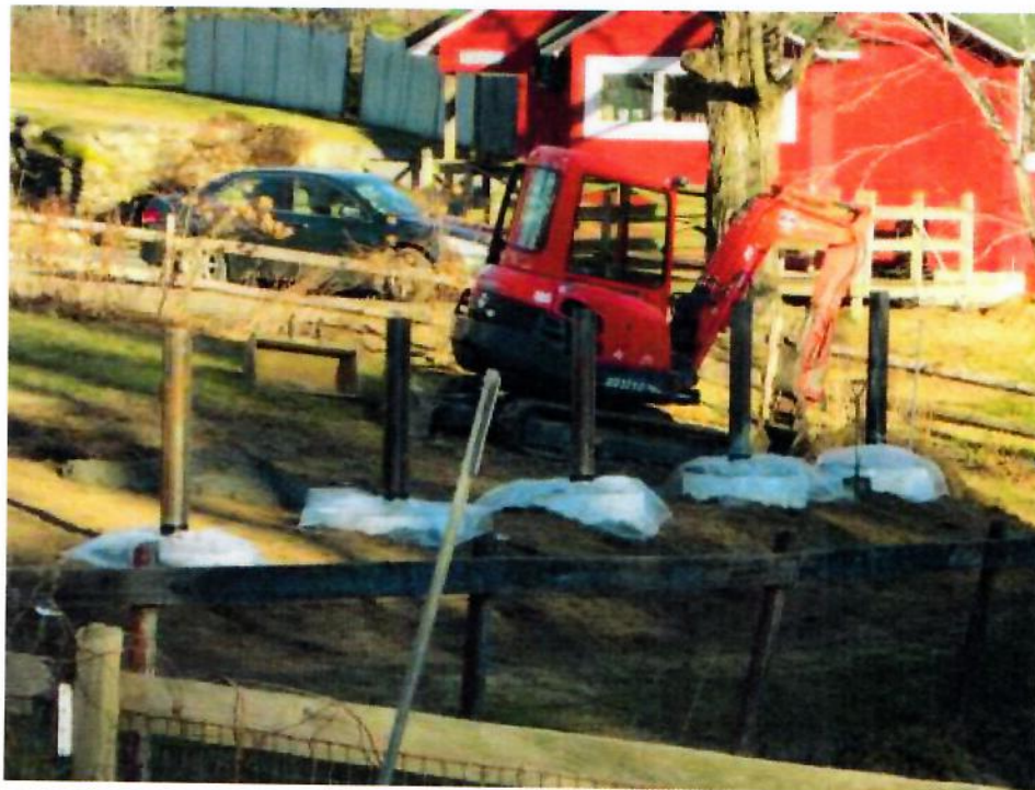
Figure 9. Direct Embedment Mounting Posts Set in Concrete.
