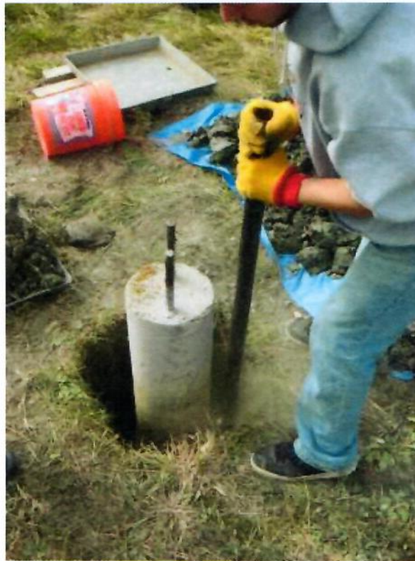
Figure 26. Placing and Tamping Backfill Around Overdrilled Pedestal Foundation.
