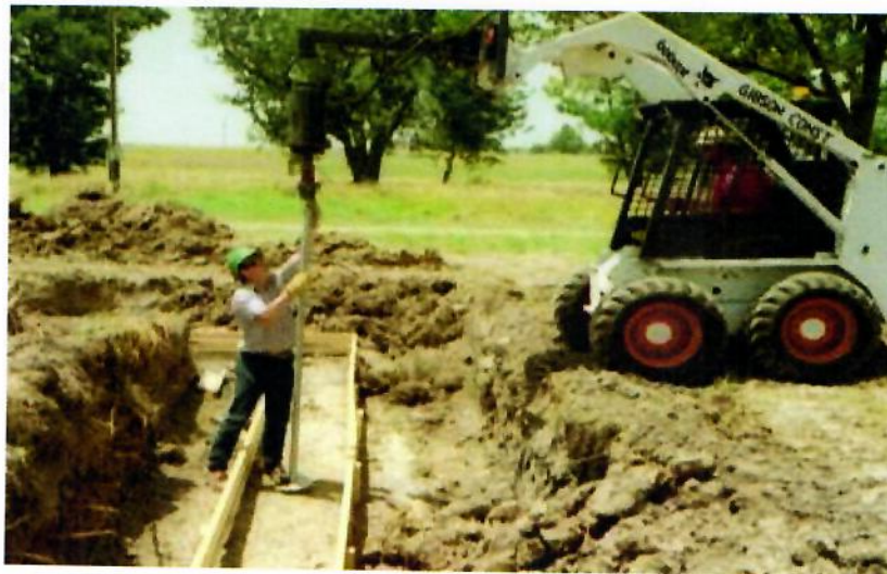
Figure 70. Using a Bobcat Loader to Install Helical Piles.
