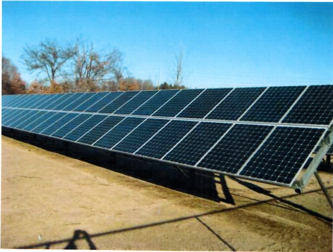
Figure 1. Typical Low-Level Ground-Mount PV Solar System. (Mountain Farms Mall – Hadley, Ma.)
