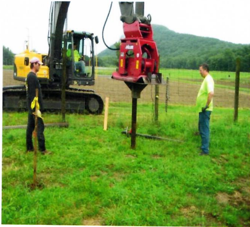
Figure 42. Using a Vibratory Plate Compactor to Install Steel Piles.
