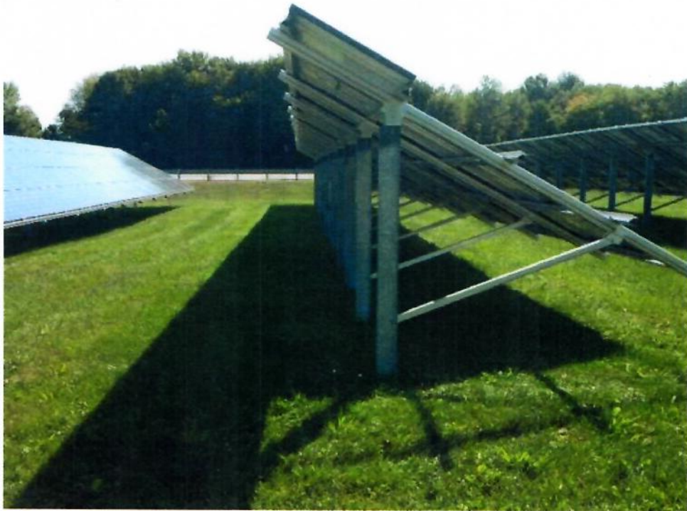
Figure 40. Driven H Piles Supporting a PV System.
