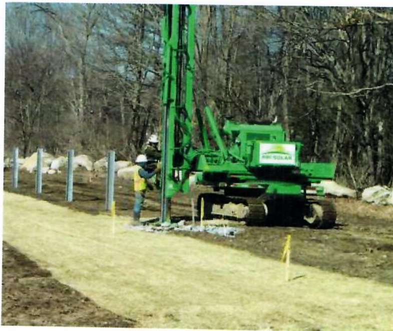
Figure 43. Commercial Installation of Steel Piles Using a Special Pile Hammer System.
