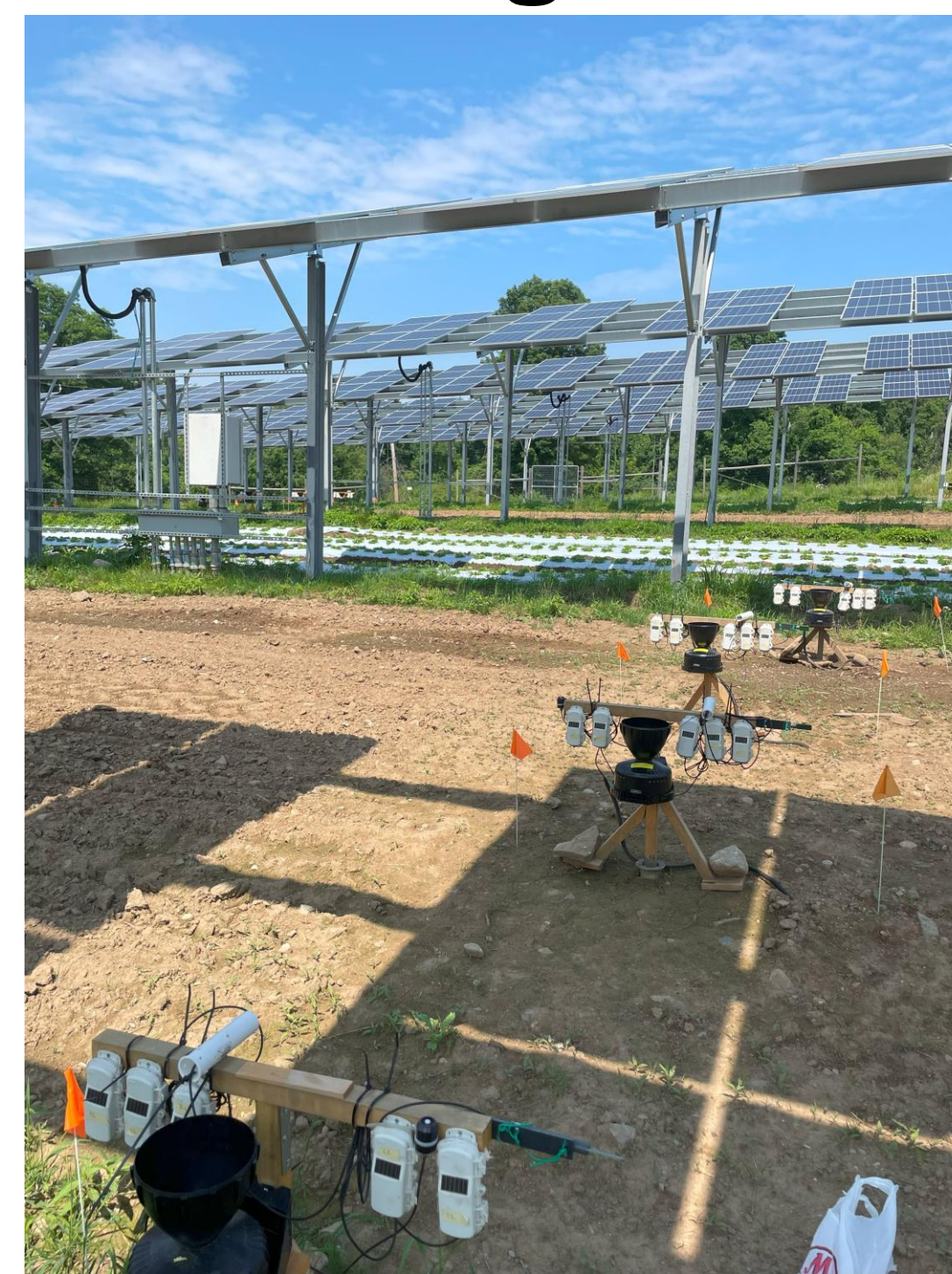
Photo 1: Array bed positions 1-4 in a bay of solar panels (6/16/23).
