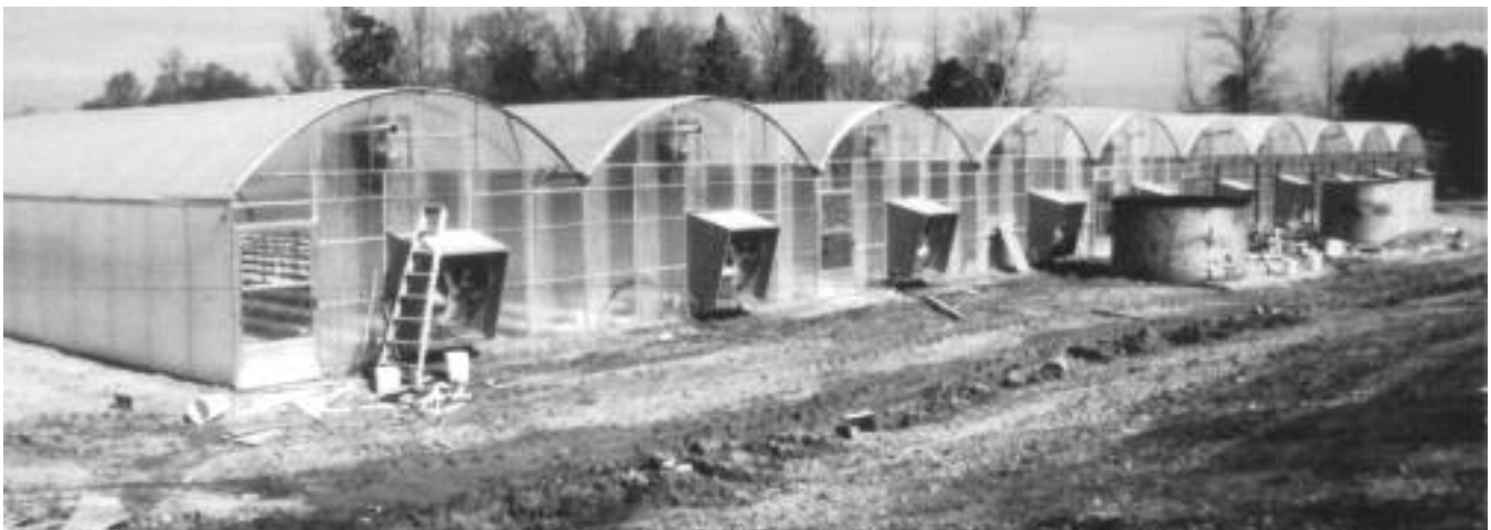
Shown are 10 greenhouse bays in a gutter-connected range (1/2 acre).
