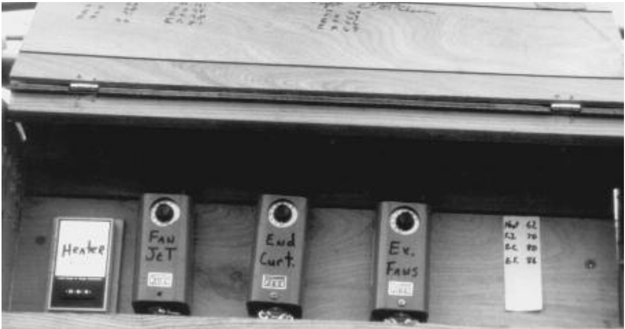
Locating thermostats in a box will avoid direct sun on them. An aspirated box is best.
